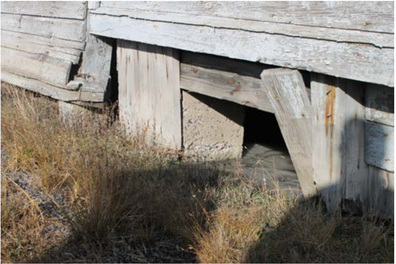
Photo 22c. Western façade of the Utica Canal Terminal showing the concrete beam foundation, facing northeast.
