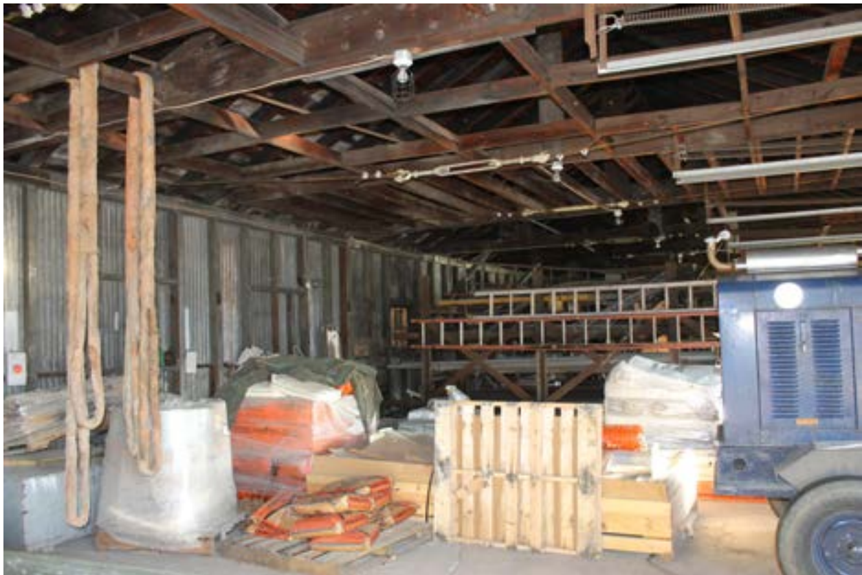
Photo 17. Interior of wood framed warehouse showing the use of cables to secure the structure.
