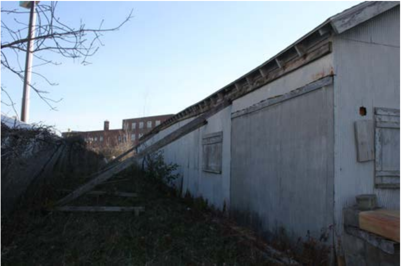
Photo 16. Wood braces along the eastern façade of the wood framed warehouse building, facing southeast.
